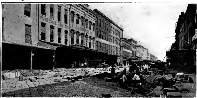
POYDRAS STREET, NEW ORLEANS, IN PROCESS OF REPAIR These heavy granite blocks were relaid as a base for the new pavement
